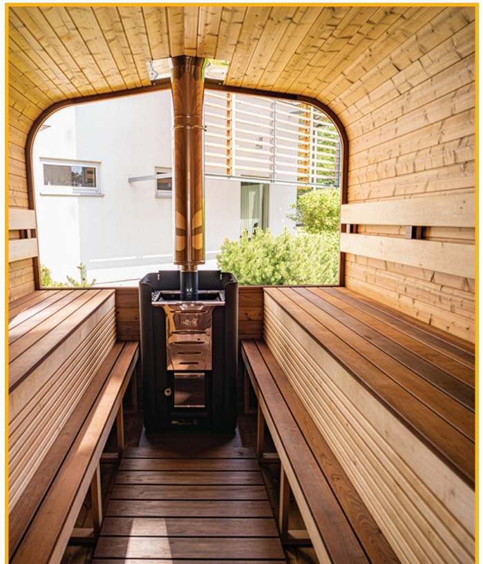
Walls: BAREL FIN / 42x115 / Thermo Pine Bench: PHL / 28x90 / Thermo Aspen
